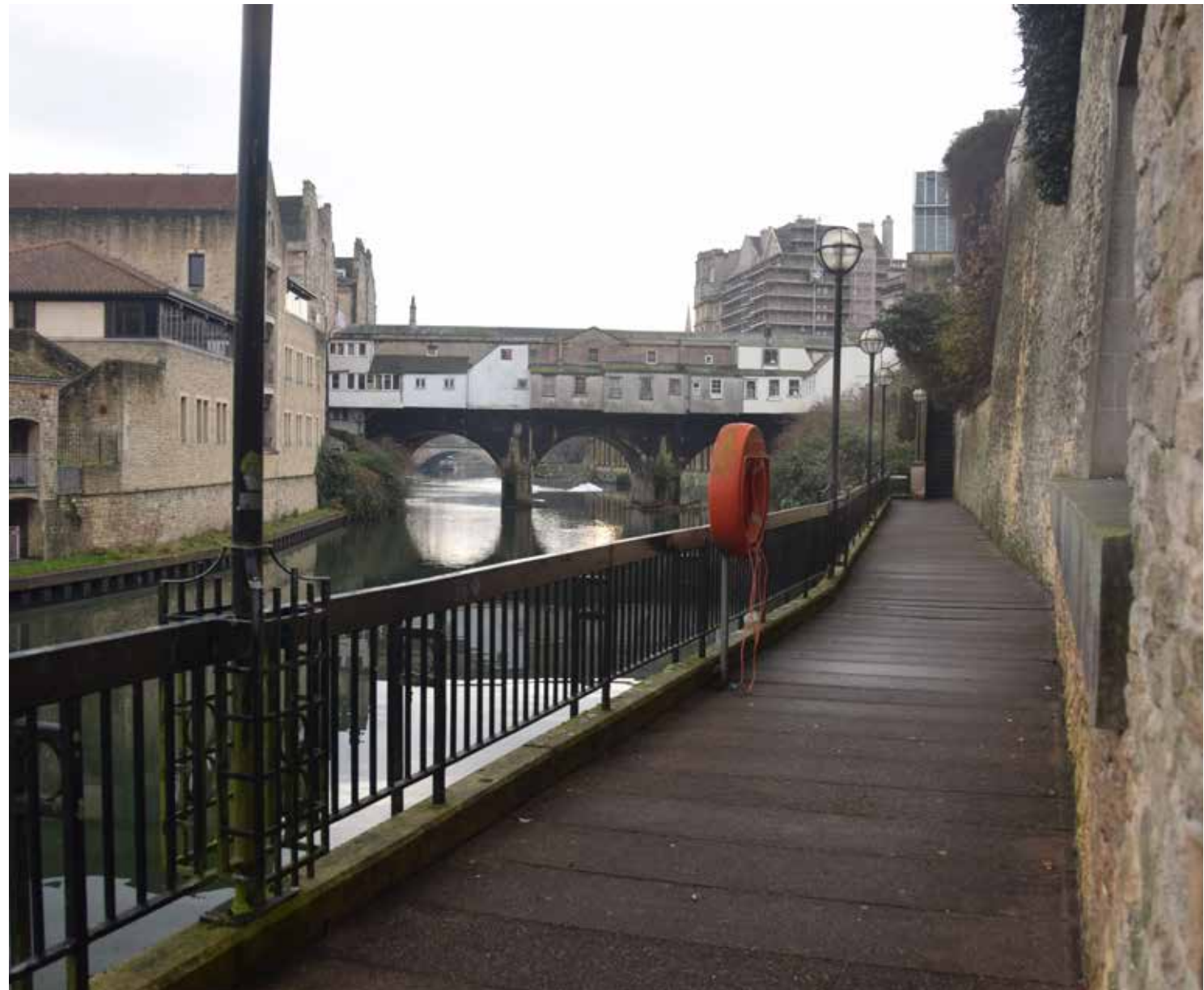
Right: Bath Podium development has established a precedent for creating new riverside connections north of Pulteney Weir.
