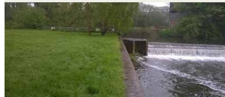
The pool and traverse fish pass on Keynsham Weir
