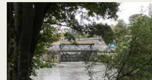
Twerton Water Level Control Gate
