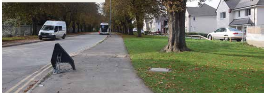
Completed Somerdale Housing Development
